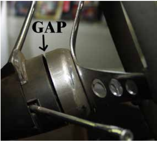
This photo shows the gap between the steering wheel hub and turn signal switch housing.
